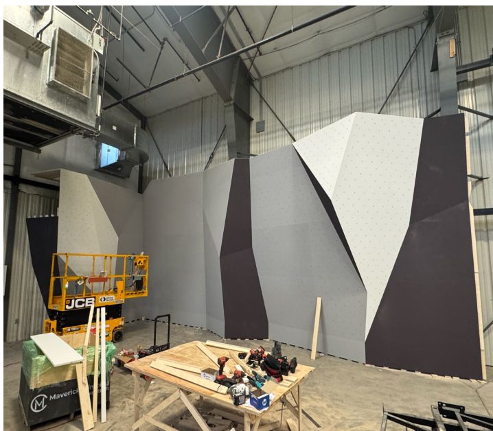
EFH Climbing Wall Progress
