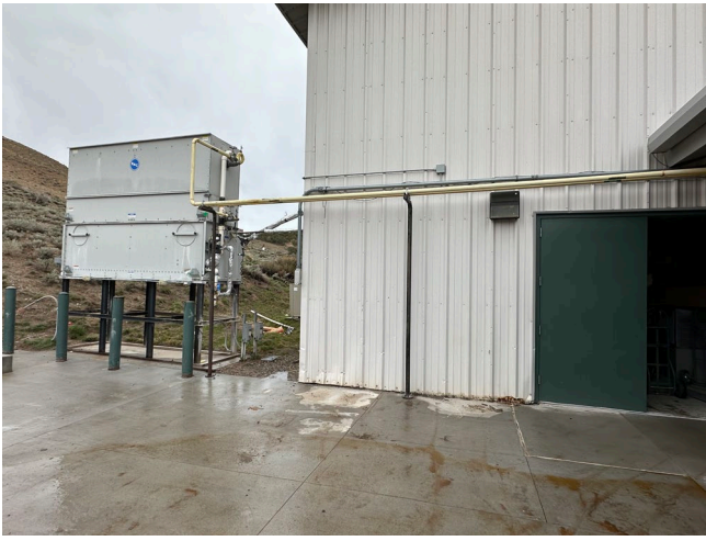
Cooling Tower – Before
